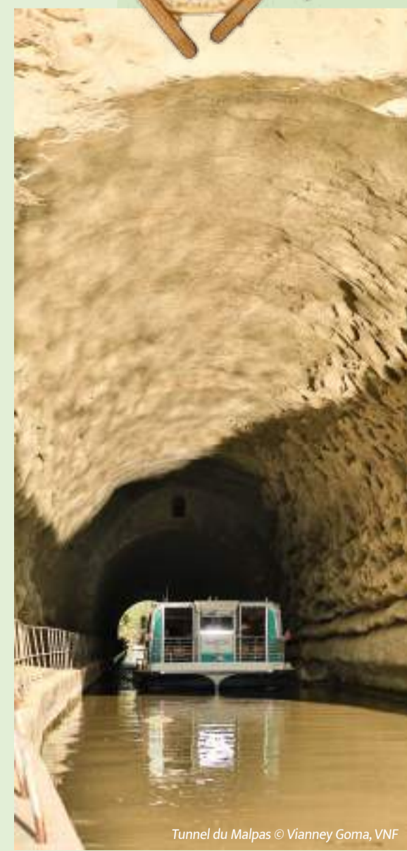
Tunnel du Malpas © Winney Gama, VNF
